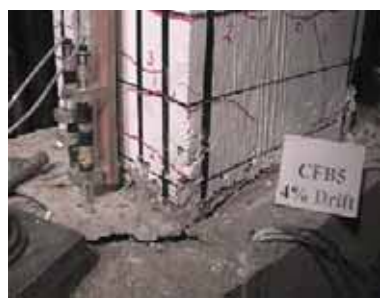
(a) Beam CFB5
