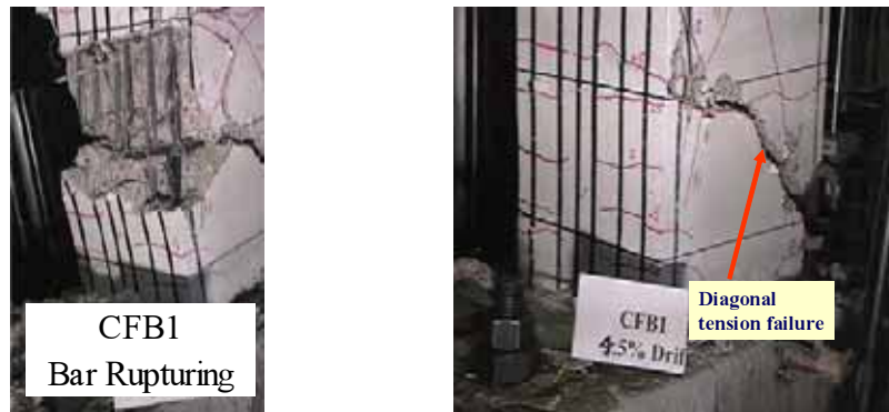
Fig.4 Observed Damages in Beam CFB1
