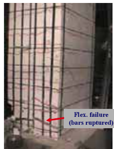
(b) Beam CFB6
