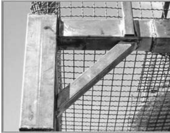
Fig.10 Using corbels for strengthening the connections
