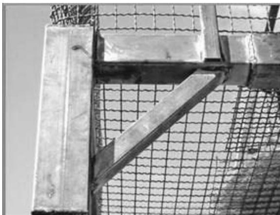
**Fig.10** Using corbels for strengthening the connections
