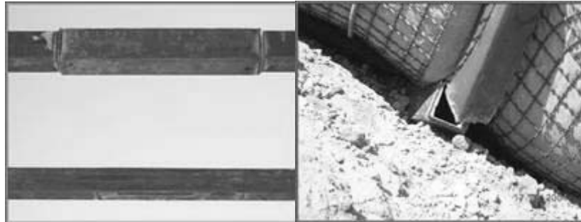
Fig.5 Welding the two ends of the stiffening box element
