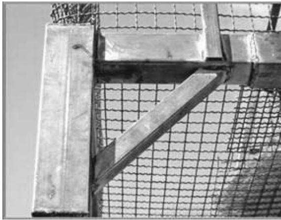
Fig.10 Using corbels for strengthening the connections
