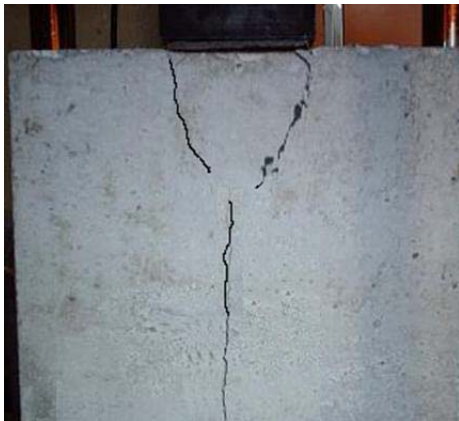
a. Crack forming
