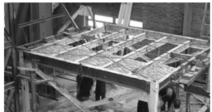
Fig. 10 Specimen-5 retrofitted by DXS on the floor under construction
