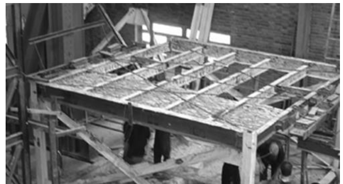
Fig. 10 Specimen-5 retrofitted by DXS on the floor under construction
