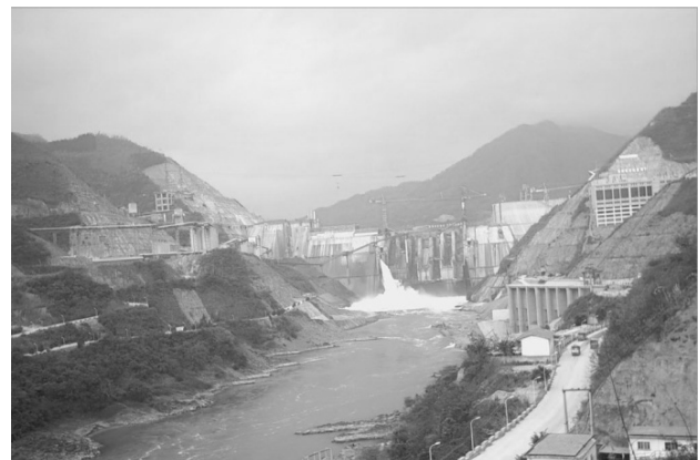
Fig. 1 Longtan hydropower station
