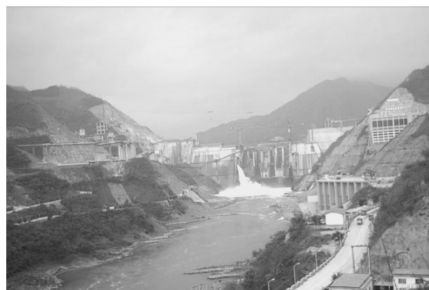
Fig. 1 Longtan hydropower station
