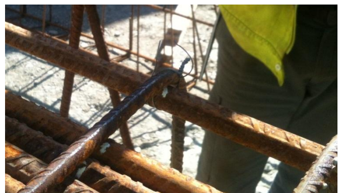
Fig. 5 Close-up of mechanical tying
