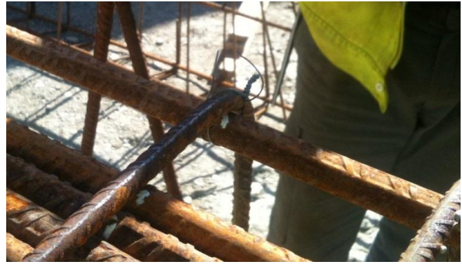
Fig. 5 Close-up of mechanical tying
