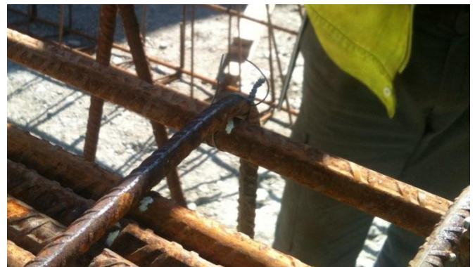
Fig. 5 Close-up of mechanical tying
