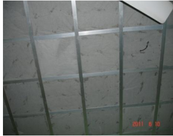
Fig. 10 Retrofitted industrial waste material false ceiling
