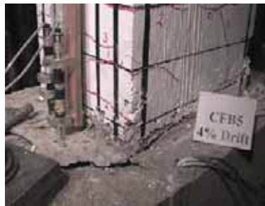
(a) Beam CFB5
