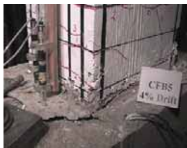
(a) Beam CFB5
