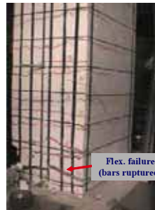
(b) Beam CFB6
