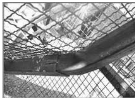
Fig.6 Changing the direction of welding
