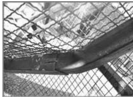
Fig.6 Changing the direction of welding
