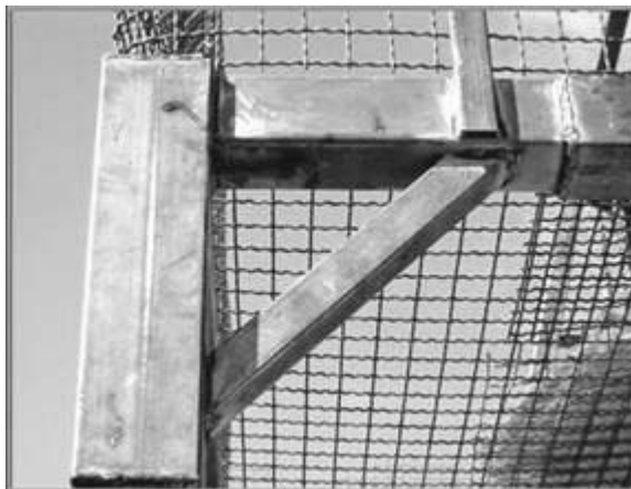
Fig.10 Using corbels for strengthening the connections
