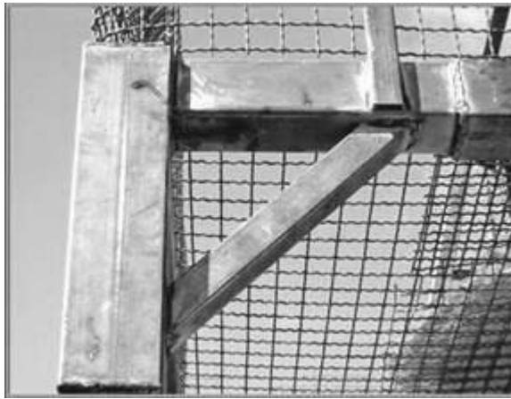
Fig.10 Using corbels for strengthening the connections
