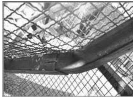
Fig.6 Changing the direction of welding
