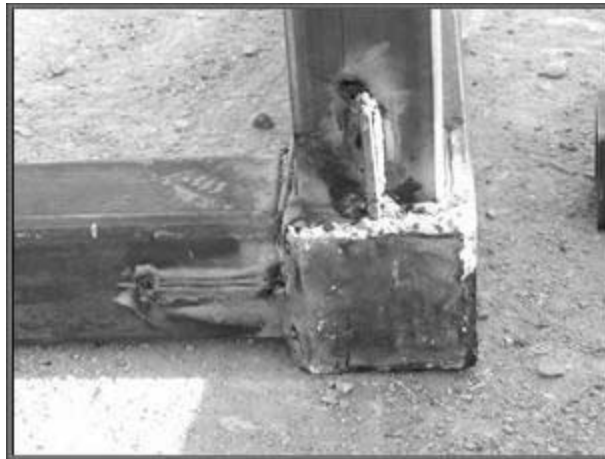
Fig.8 Using end plates and dowel plates in beam to column moment connections
