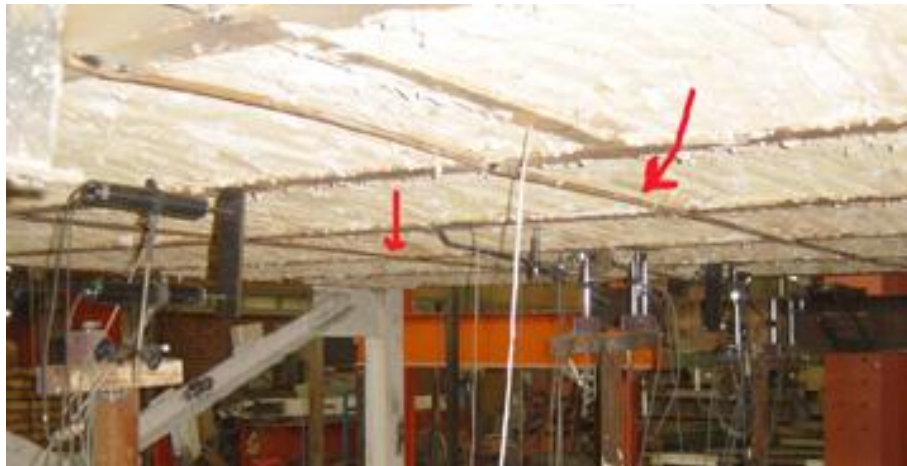
Fig. 17 Two parallel rods welded below the jack arch slab in specimen 3 reduced the widening between two adjacent joists
