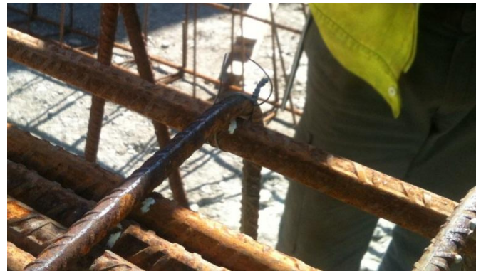
Fig. 5 Close-up of mechanical tying
