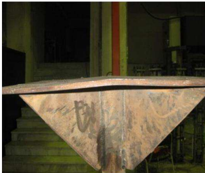
Fig. 25 Sagged plate near the connecting bolt
