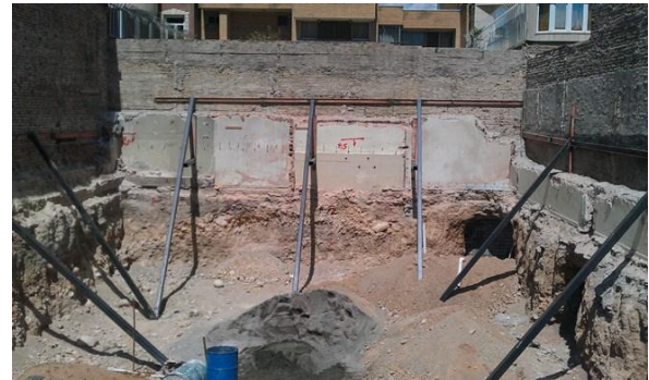
Fig. 7 Photo of excavation
