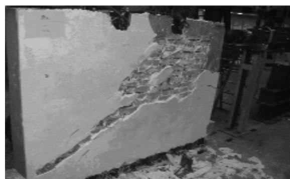
Fig 13 Separation of plaster due to crack formation in specimen B at last loading step
