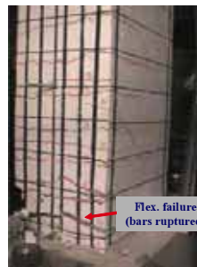
(b) Beam CFB6
