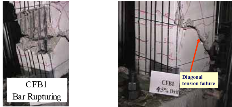
Fig.4 Observed Damages in Beam CFB1
