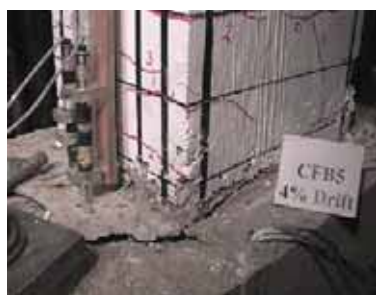
(a) Beam CFB5
