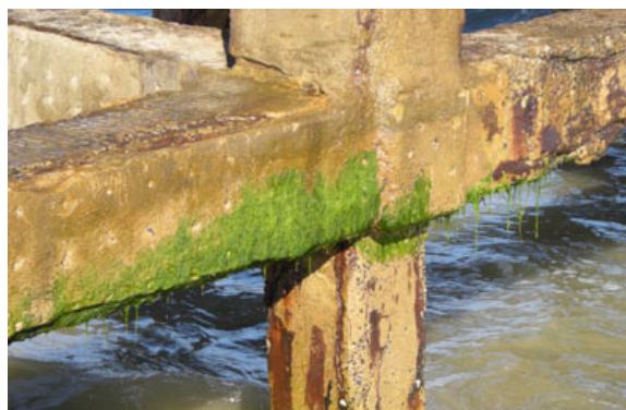
Fig.1. Growth of Marine Seaweed on Structural Components
