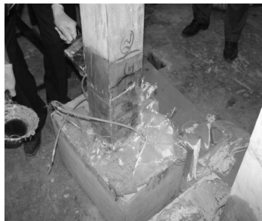
Fig.9 Installation of prefabricated composit sheets
