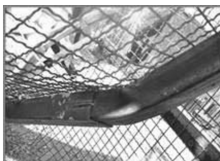
Fig.6 Changing the direction of welding
