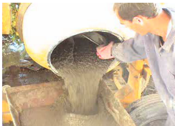
Fig. 1. Mixing of SCLWC
