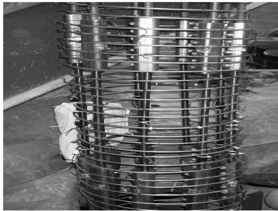
Fig. 1. SMA bars connected to steel bars
