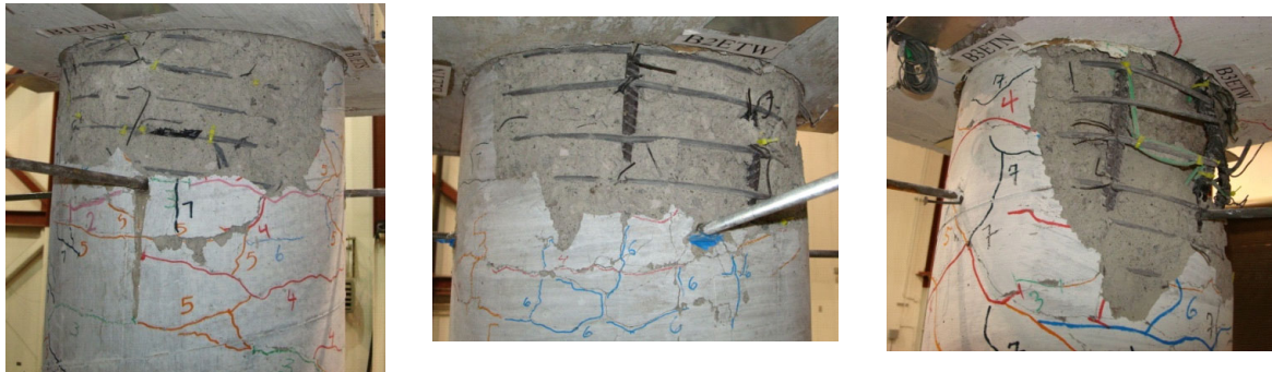
Fig. 7. Upper plastic hinge after final motion: left to right, SMA pier, PT pier, and ISO pier
