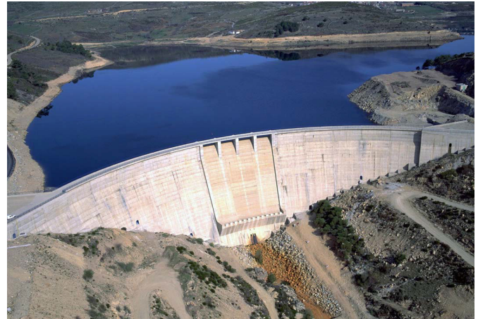
Fig. 1 La Aceña dam (Central Spain). General view
