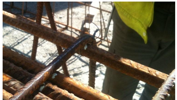
Fig. 5 Close-up of mechanical tying
