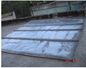
Fig. 9 Retrofitted expanded polystyrene with saw dust and aluminum sheet
