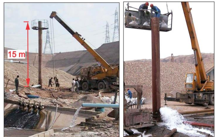
Fig. 5 (Left): controlling the artesian flows by adding long vertical pipes at the top of the relief wells at the Karkheh dam site. (Right): placing filter materials after controlling of the artesian flow
