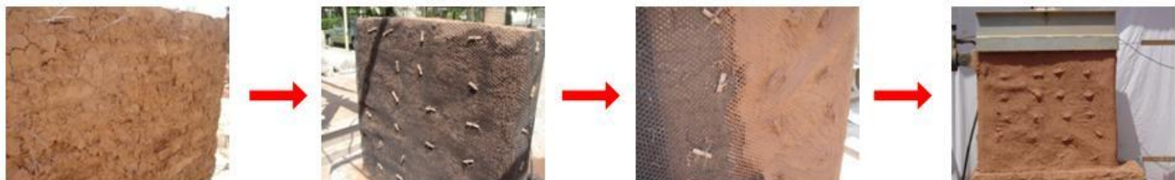
Fig. 14 Installation process of polypropylene lace on adobe walls
