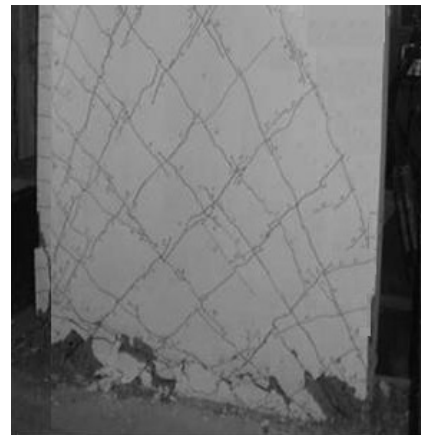
Fig.16. Experimentally established failure mode of a typical shear wall (shear wall 4-1750/1.00).
