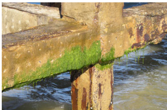
Fig.1. Growth of Marine Seaweed on Structural Components
