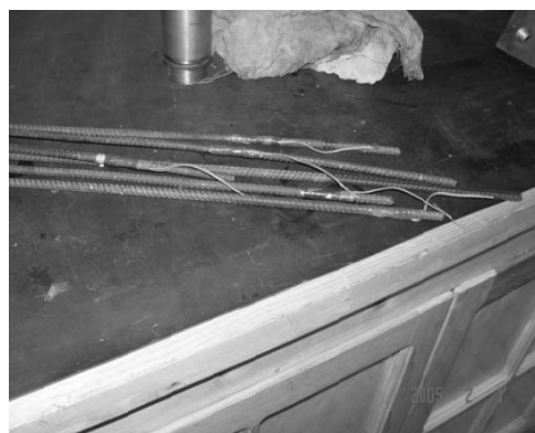
Fig.4 Strain gauges were installed on the bars
