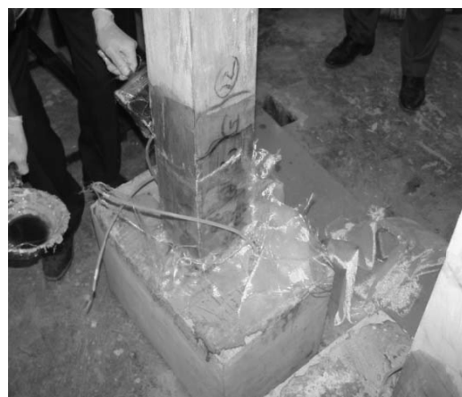
Fig.9 Installation of prefabricated composit sheets
