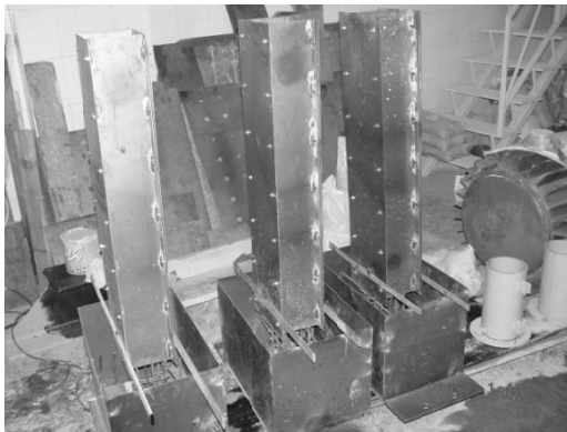
Fig.3 Specimens reinforcing cage in their formworks
