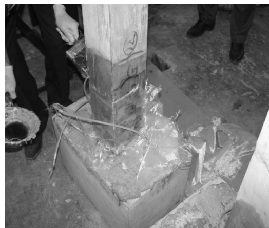
Fig.9 Installation of prefabricated composit sheets
