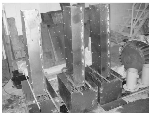
Fig.3 Specimens reinforcing cage in their formworks
