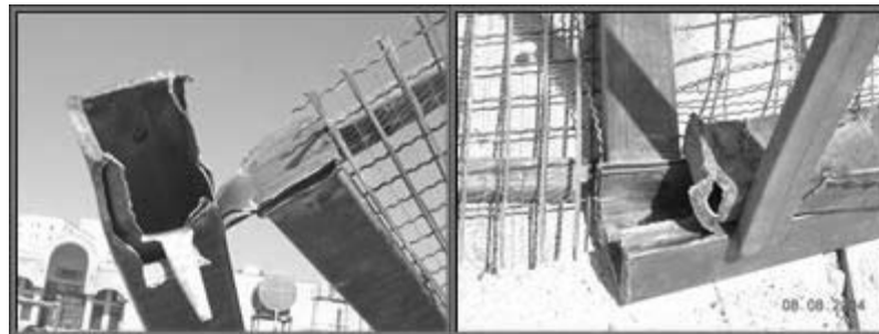
Fig.7 Destruction of beam to column moment connection
