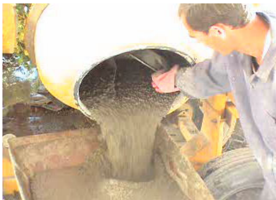
Fig. 1. Mixing of SCLWC
