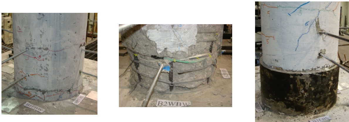
Fig. 8. Lower plastic hinge after final motion: left to right, SMA pier, PT pier, and ISO pier
