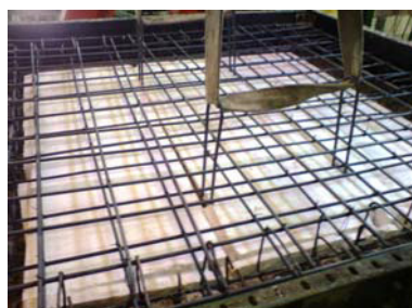
c) Slab reinforcement and hanging support
