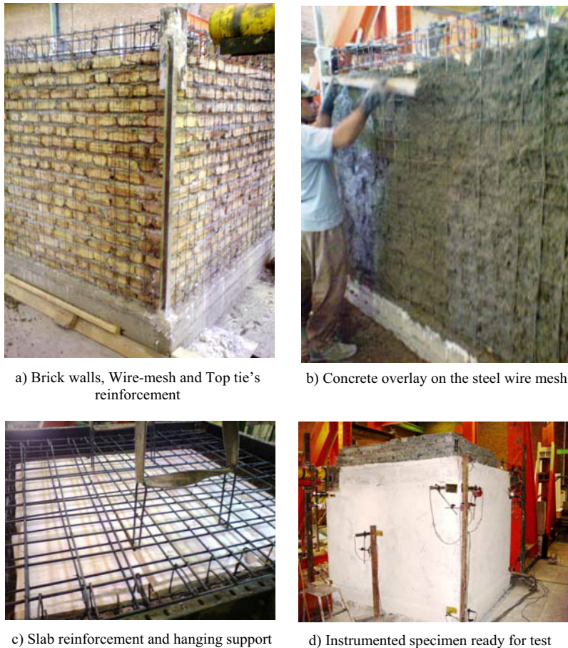
Fig. 4. Making Specimen SUBB ready for test
