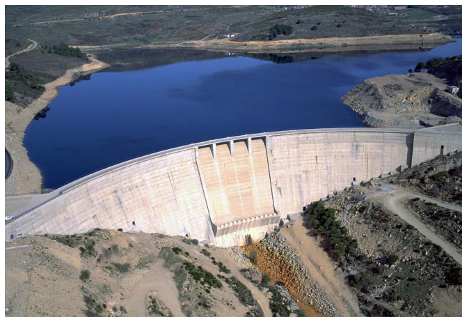
Fig. 1 La Aceña dam (Central Spain). General view
