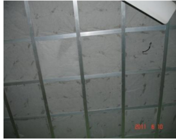
Fig. 10 Retrofitted industrial waste material false ceiling
