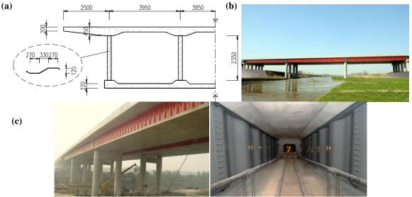
**Fig.1** Exemplified bridge structure with corrugated webs completed in China, 2010: (a) cross-section of a box girder with corrugated webs (dimensions in mm), (b) overview of the bridge, (c) details of corrugated steel webs jointing flange plates [2,3]
