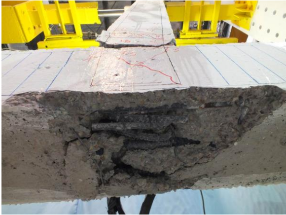
Fig. 9 Crushed concrete of panel zone in specimen WR at the end of test
