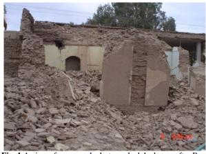
Fig. 1 A view of one sample destroyed adobe house after Bam earthquake
