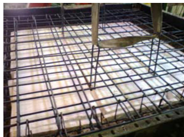
c) Slab reinforcement and hanging support
