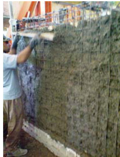
b) Concrete overlay on the steel wire mesh
