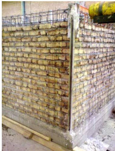
a) Brick walls, Wire-mesh and Top tie's reinforcement
